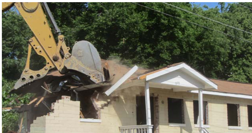
Demolition of a House on Moore Street in May of 2012
