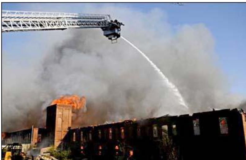
Fire in Action: Macon Firefighters work to suppress a massive fire tht would eventually destroy in the Historic Atlantic Cotton Mill.
