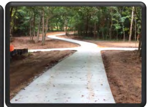
Amerson Park Sidewalk Improvements
