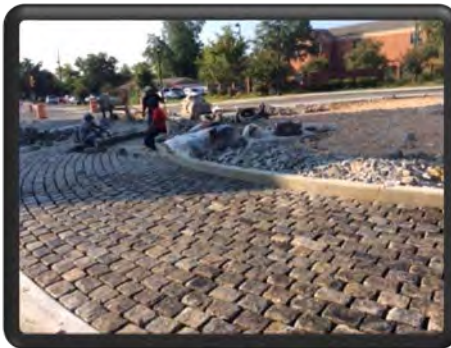
Crews use recycled cobblestones on new roundabout
