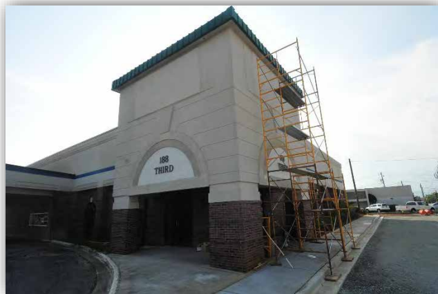
Construction on the outside of the new Tax Commissioner's Center
