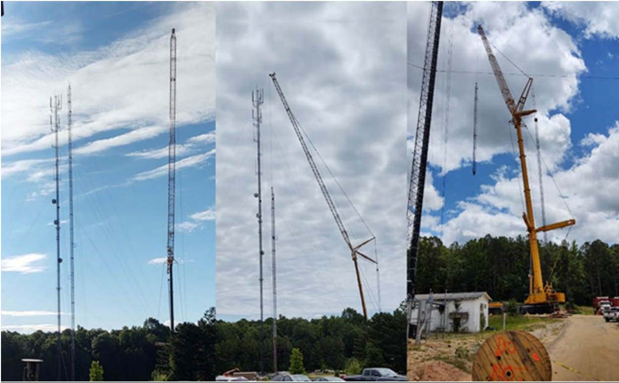
Call Center Motorola Radio Frame Removal
