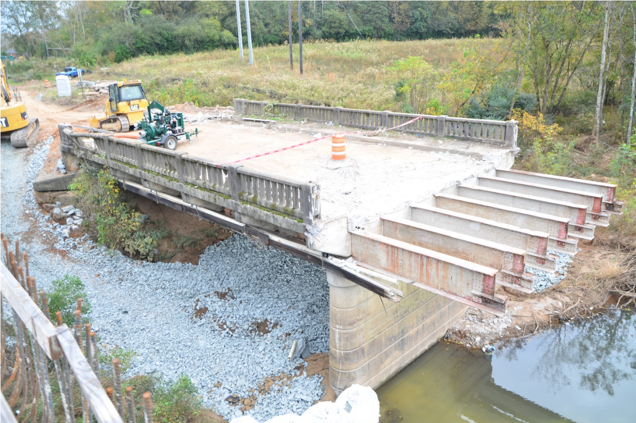
Jeffersonville Road Phase 1 Construction
