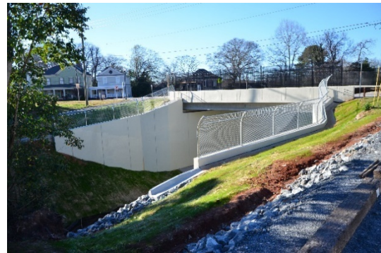
Railroad Bridge at College Street
