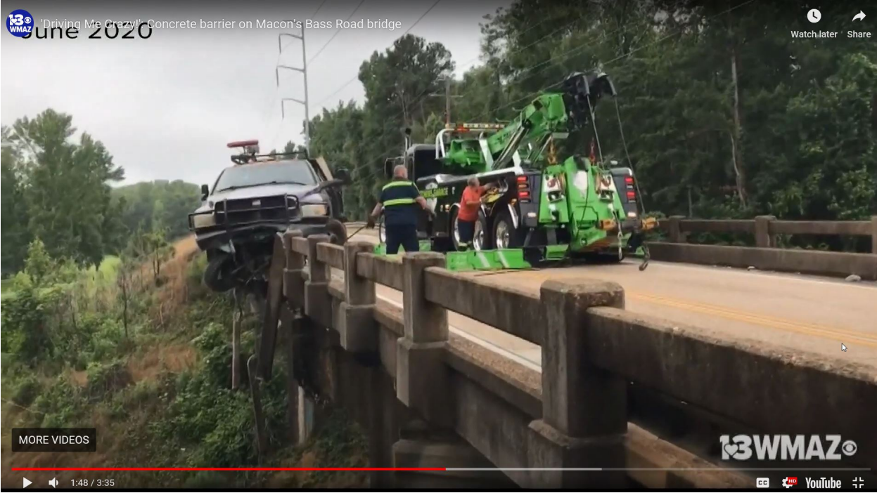
Bass Road Bridge over Railroad Damaged and Repaired
