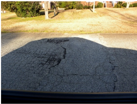
Water Wheel Court before resurfacing
