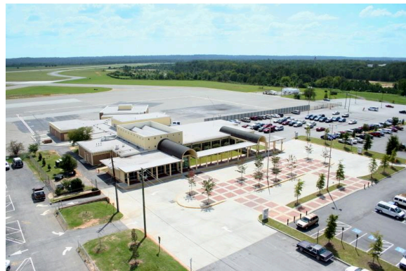
Middle Georgia Regional Airport
