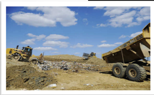
Employees covering refuse at the City of Macon Landfill
