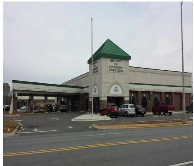
New Tax Commissioner Service Center located at 188 Third St.
