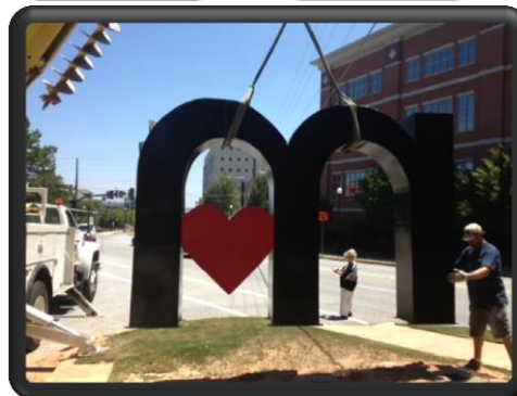
Installation of the "I Love Macon" Sign
