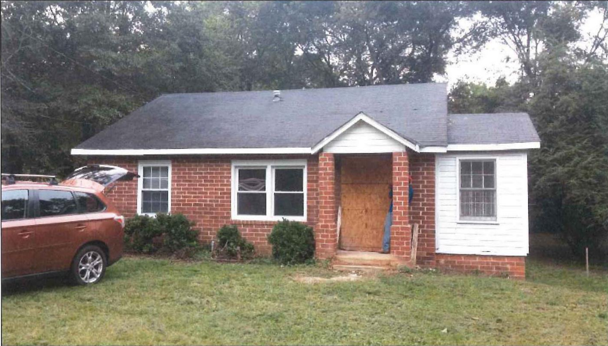
1548 Jeffersonville Road Project No. 5240-06 Parcel 32A
